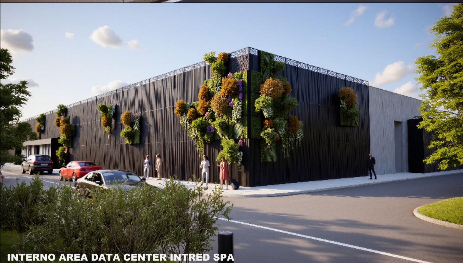
INTERNO AREA DATA CENTER INTRED SPA
