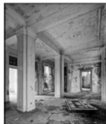
View interior of factory with column
