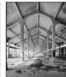
View interior of factory
